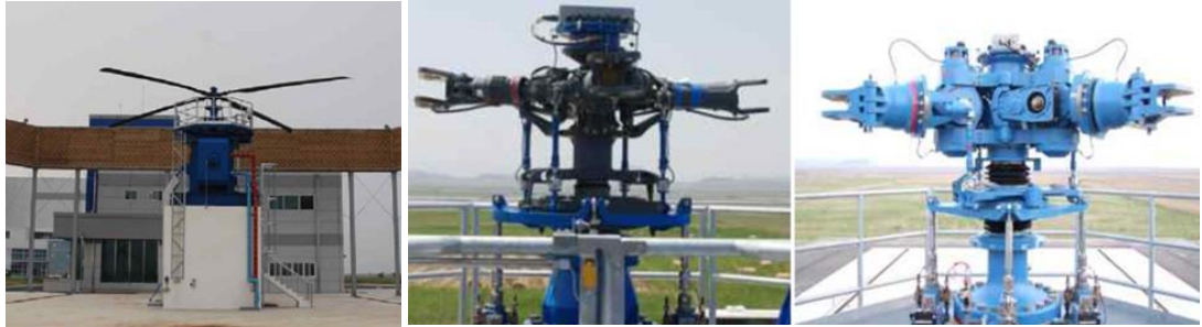
Fig. 2. KARI Whirl Tower Test Facility (WTTF)
